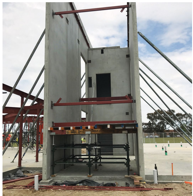
Tilt slabs are erected on the site of the new building
